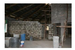
We are now focusing on completing the roof. We are also completing the inside walls. And we have started installing the electrical conduits.
